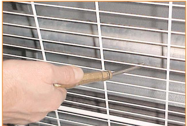
Brush away any dust on the exterior of the radiant tubes.
