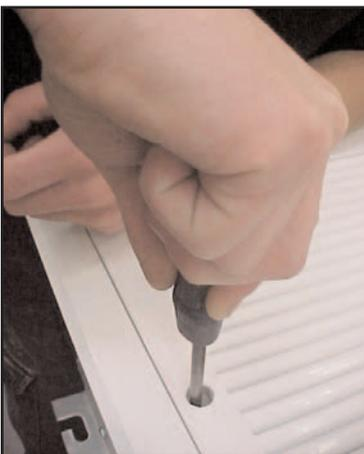
Using a pozidrive screwdriver remove the M5 screws through the access hole. To facilitate re-fitting of the grille the screws are circa 50mm long, hence multiple turns of the screwdriver will be required. The grille assembly can now be removed from the case to allow fitting of the product in the ceiling recess.
