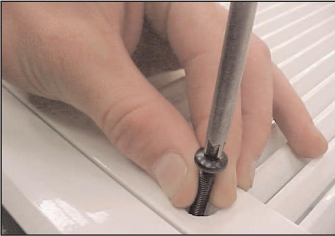
After fitting the product in the ceiling recess and adjusting the height to ensure that the grille sits flush to the ceiling (when re-fitted) take the grille assembly and refit using the two screws removed during Step 2. Snap the grommets removed in Step 1 back in place to cover the access holes.
